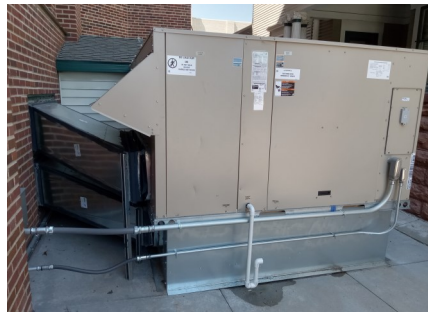
New unit with ductwork to building
