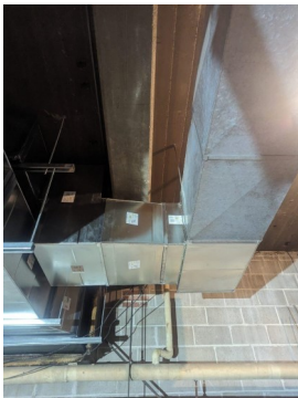
New ductwork connecting to existing inside
